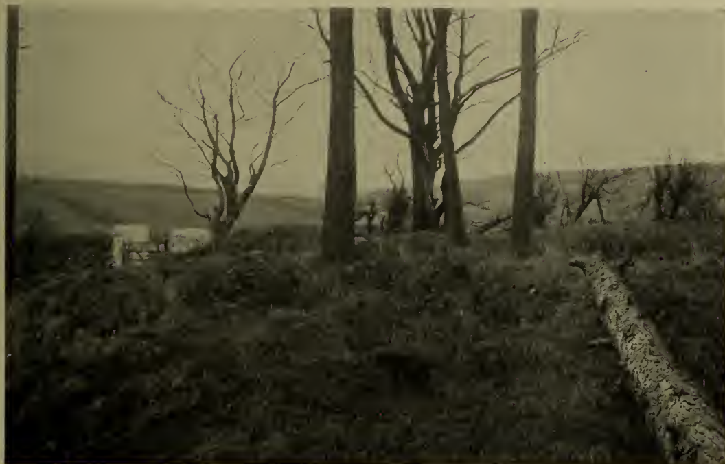
FIG. 3—FOUNDATIONS OF KEEIL, BALLAQUINNEY, MAROWN.
